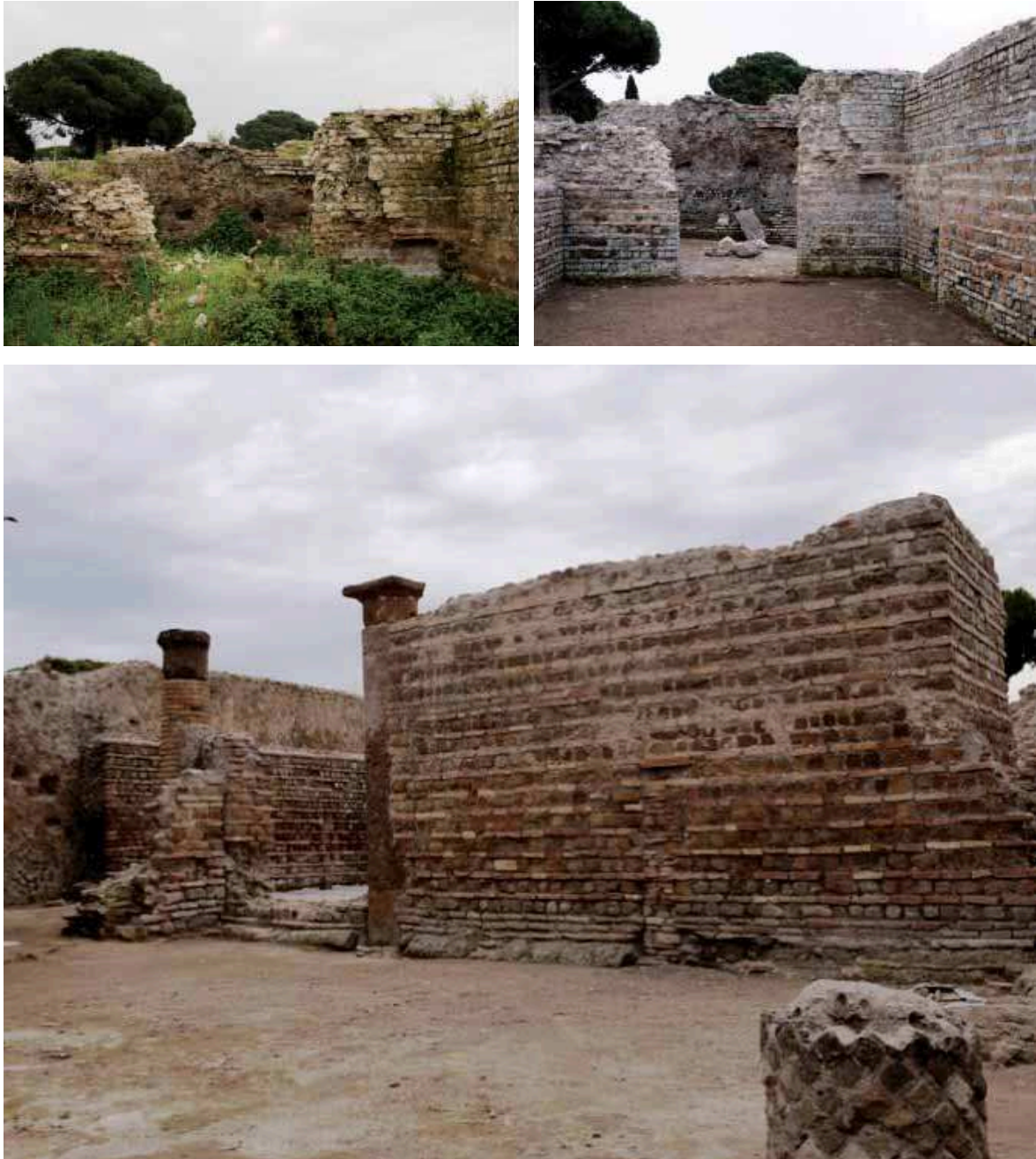
Fig.5 - A view of east side before and after restoration works; a view after restoration works
