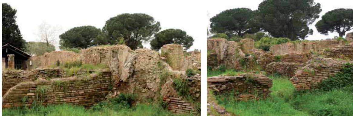
Fig.3 - Views of west side before restoration works
