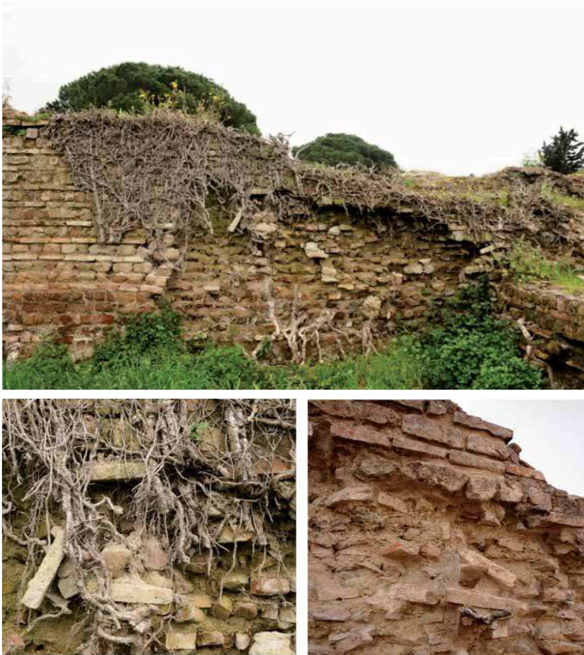
Fig.4 - Plants constitute one of the main conservative problems: restoration treatment include their gradual cutting and removal without causing further damage while this operation is carried out. In some points remains of stems incorporated in the wall structure were maintained for static reasons; East side wall detail before and after restoration works
